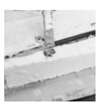
6.) Before reinstalling the cooling unit, it is necessary to put thermal mastic onto the evaporator tube.
